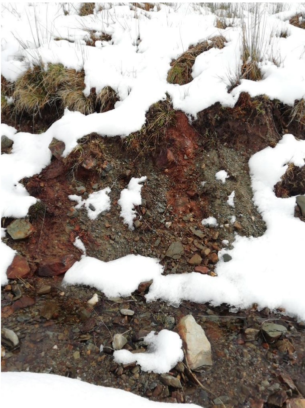
Figure 5. Gleann Casaig: signs of poor revegetation and erosion of new track slopes; viewpoint 20
