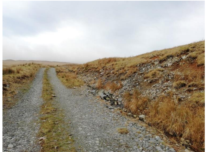
Figure 15. Derrydarroch: central verge well vegetated. To the right, the slope is visibly scarred and vegetation is pocketed; viewpoint 23
